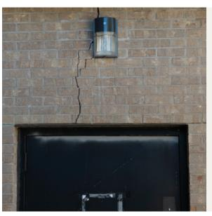
Fairview Armory: structural cracking and deterioration
