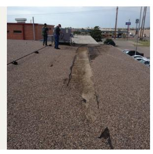
Hondo Pass Armory: roof structural failure
