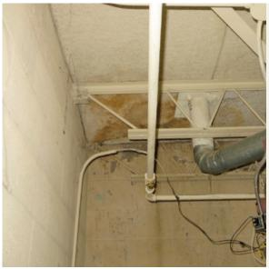
Denison Armory: roof lead and ceiling deterioration
